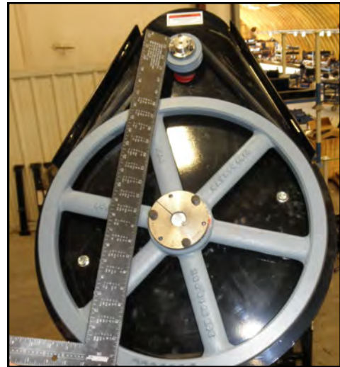
Lay a straightedge across pulley faces
