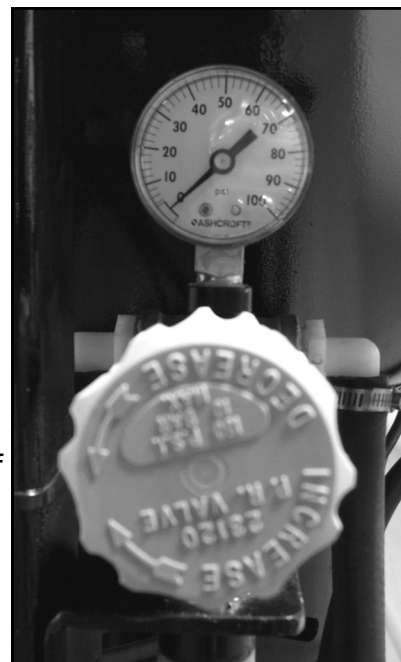
Pressure Gauge and Regulator
