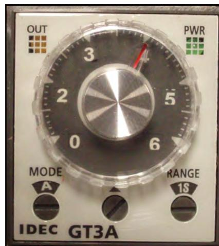
**B. Slide Gate Delay Open Timer:** Connected in conjunction with the AUTO STARTUP button and the lower proximity switch. When the AUTO STARTUP button has been pressed, this timer will begin timing down. Once the timer has timed out, the slide gate will open, sending seed down through the atomizer. This timer gives the pump(s) a head start before seed is introduced. The timer is set to Mode "A".
