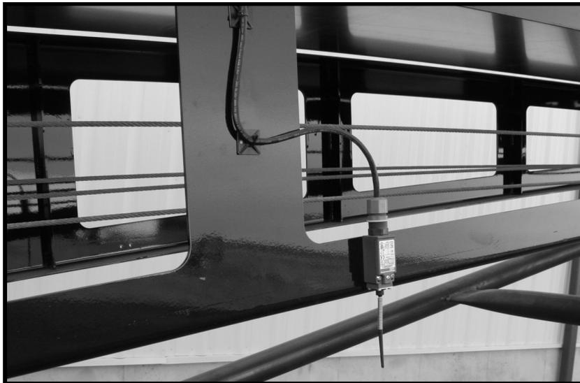
Picture of the limit switch after installation.
