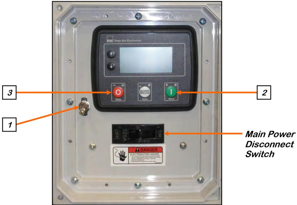
**STEP 1 - Turn On Panel Display:** Move the control panel power switch up into the ON position. The display will turn on and the red LED on the start switch will begin to flash on and off. The icon in the lower right corner indicates what mode of manual operation the generator is in. See table below.
