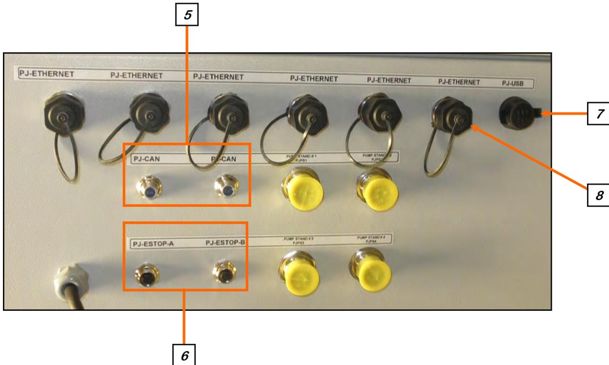
9. Connect the 19 pin yellow cable from PJ6012 on the Tri-Flo ® control panel to the shielded junction box located next the distribution spout.
