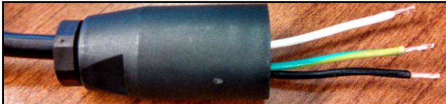
3. Wire motor leads into the correct terminations per your schematic. For USC pump motors, 1 = Ground, 2 = White, and 3 = Black.
