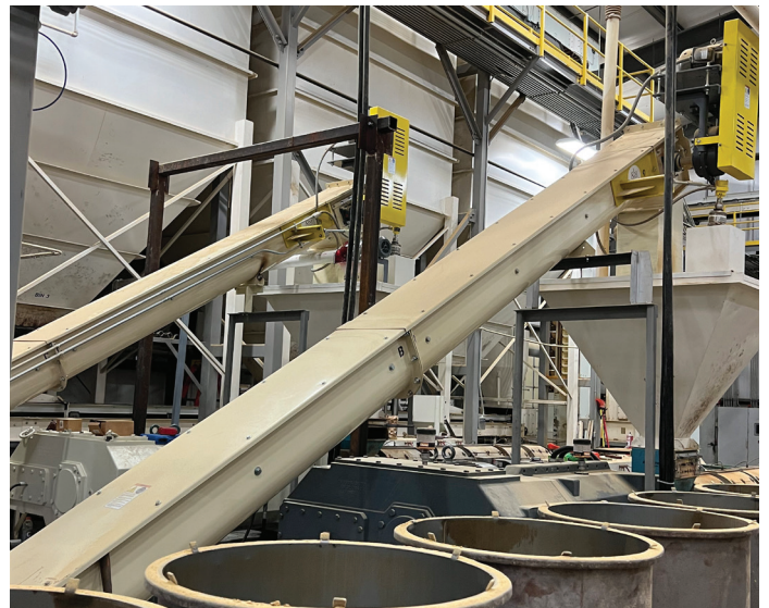
INCLINE RB CONVEYOR
